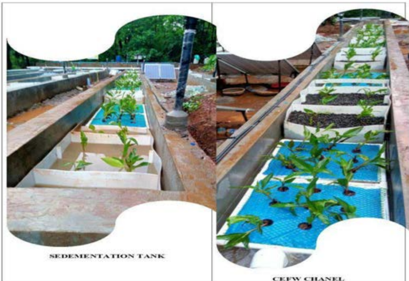
IMAGE 17 : PHOTOGRAPHS OF FLOATING RAFTERS OF 1MLD IN-SITU TREATMENT PROJECT
