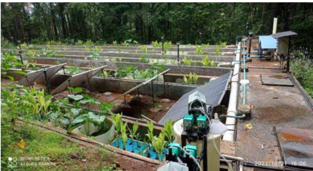
IMAGE 11 : SITE PHOTOGRAPHS OF 1MLD IN-SITU TREATMENT PROJECT
