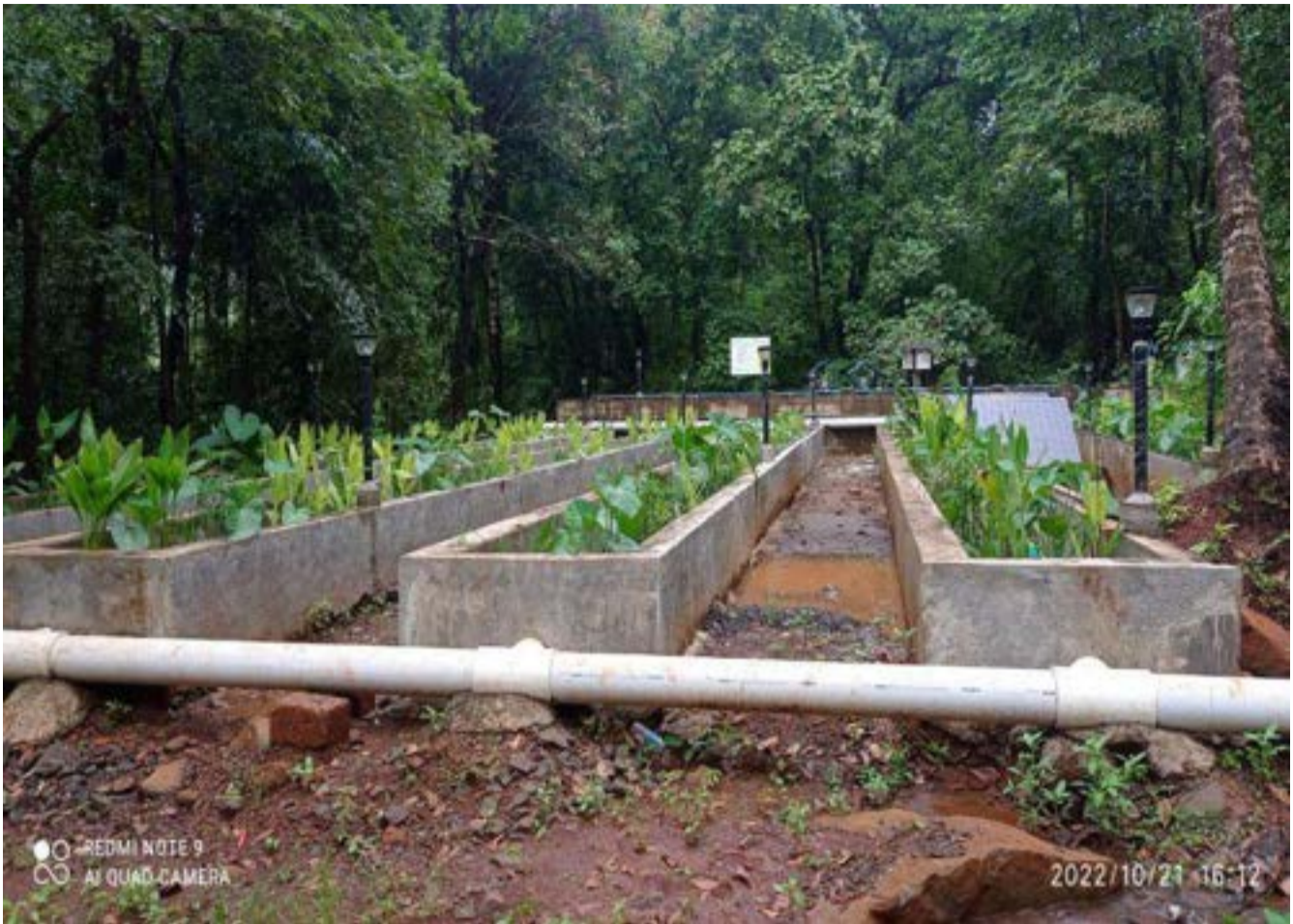
IMAGE 12 : SITE PHOTOGRAPHS OF 1MLD IN-SITU TREATMENT PROJECT
