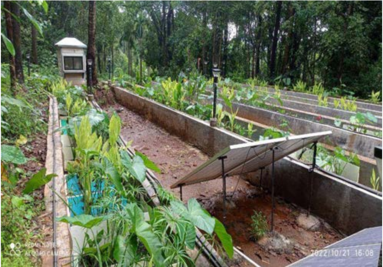
IMAGE 13 : SITE PHOTOGRAPHS OF 1MLD IN-SITU TREATMENT PROJECT
